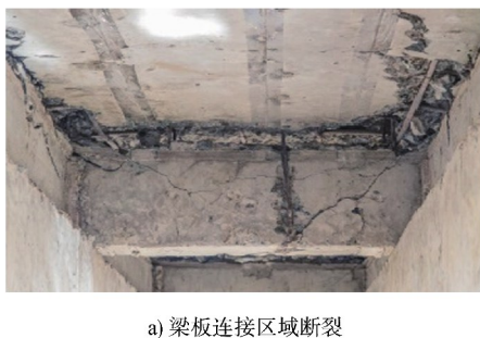
图9 空中爆炸荷载作用下的RC梁破坏效应 Fig.9 Failure effects of RC beam under air explosion
