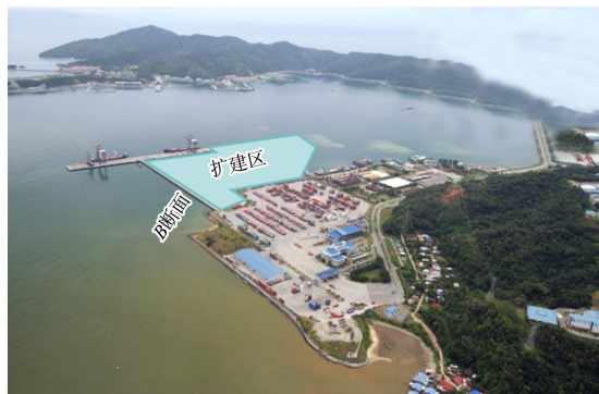
图1 马来西亚沙巴湾杂货码头现状 Fig.1 Current situation of Sabah Bay grocery terminal in Malaysia
