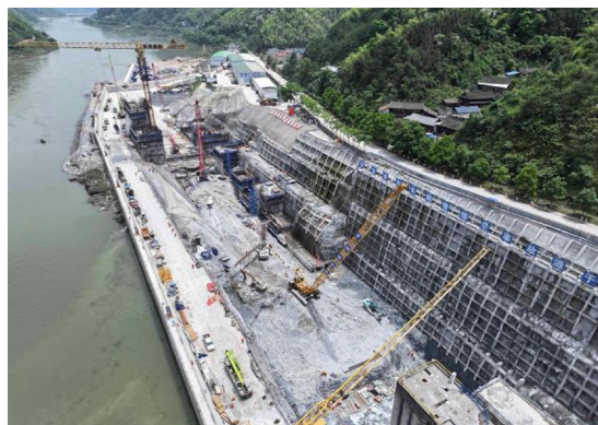
图 13 洪江船闸边坡支护完成状态 Fig. 13 Completion status of slope support of Hongjiang Ship Lock
