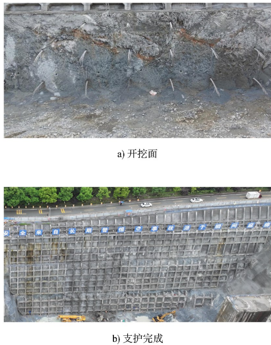
图 8 右边坡 B-1/1、B-1/2 开挖面及支护完成状态 Fig. 8 Excavation face and support completion status of right slope B-1/1 and B-1/2
